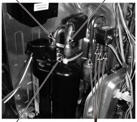
Discharge temperature thermistor Brazed parts of 4-way valve
